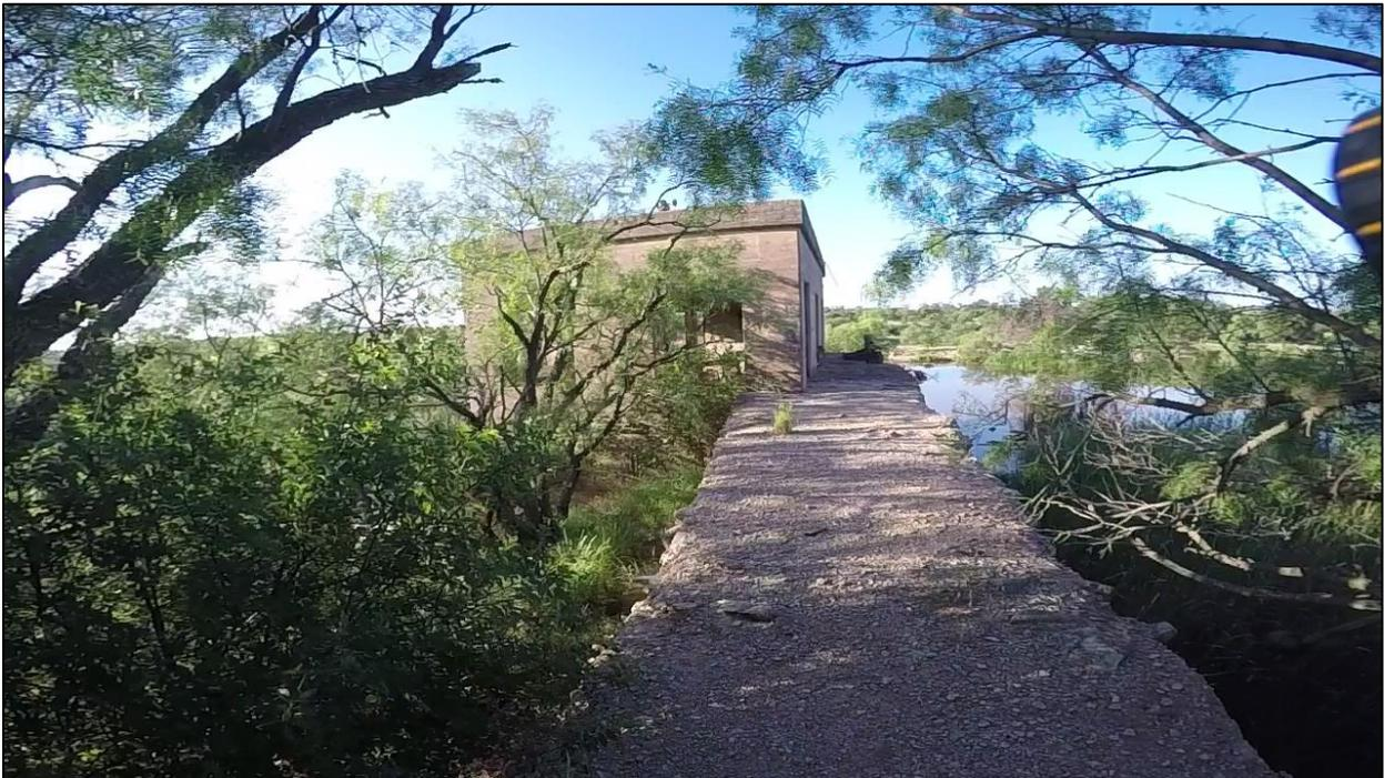
Figure 28. Overview of concrete dam where it adjoins the earthen levee, looking south out to lake and pumphouse.
