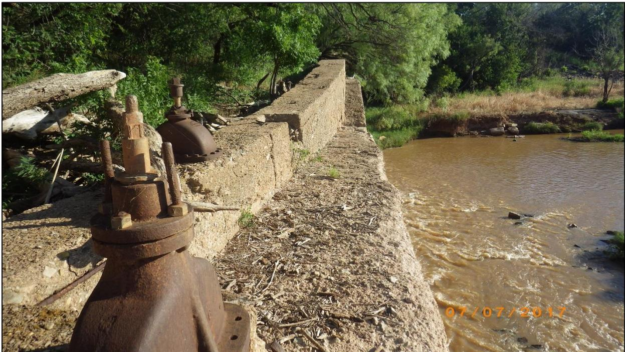
Figure 32. Overview of dam wall extending north from pumphouse. The pipeline from the pumphouse appears to be on top the dam and extends towards the intake structure.
