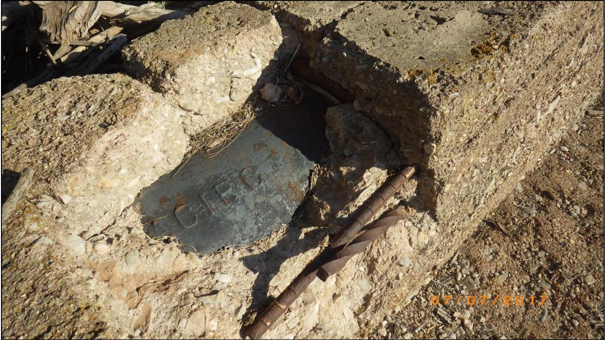
Figure 33. View of broken concrete exposing pipe and two kinds of rebar. Damascus Twist Rebar is present in the structure.
